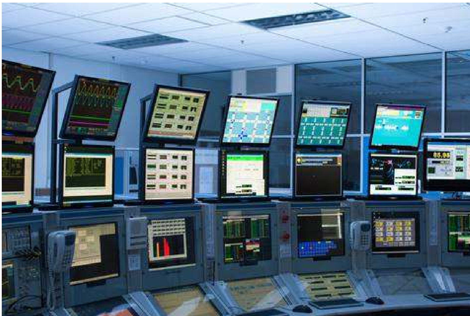
Development of SCADA-based industrial automation applications
